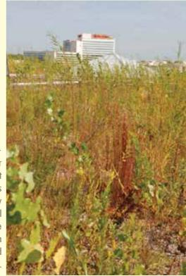
Green roofs are another storm water treatment method which replicates natural processes by absorbing rain fall and returning it to the atmosphere through evaporation and transpiration.
